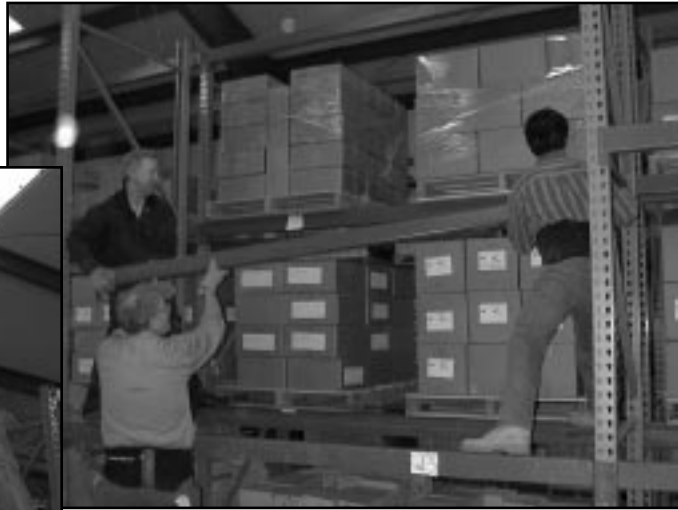
Assembling the storage racks
