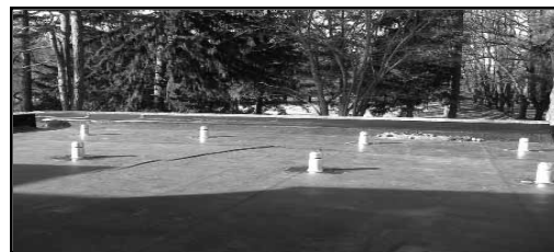
BIBLE HOUSE ROOF ABOVE KITCHEN AREA
